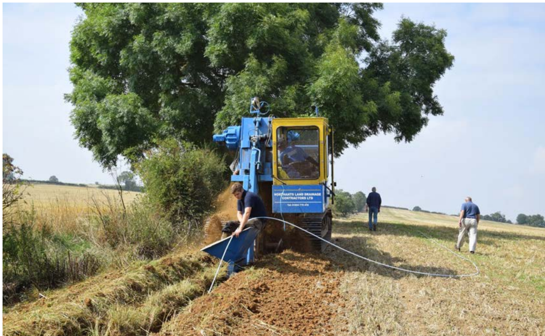
Laying broadband cable in Tove Valley
